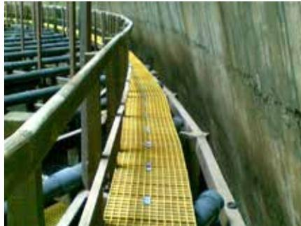
Standard Moulded FRP Grating Type 13 used as an anti-slip open mesh topping for existing structure
