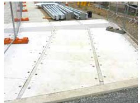
Slabs can be cut on site or in factory to suit exact dimensions
