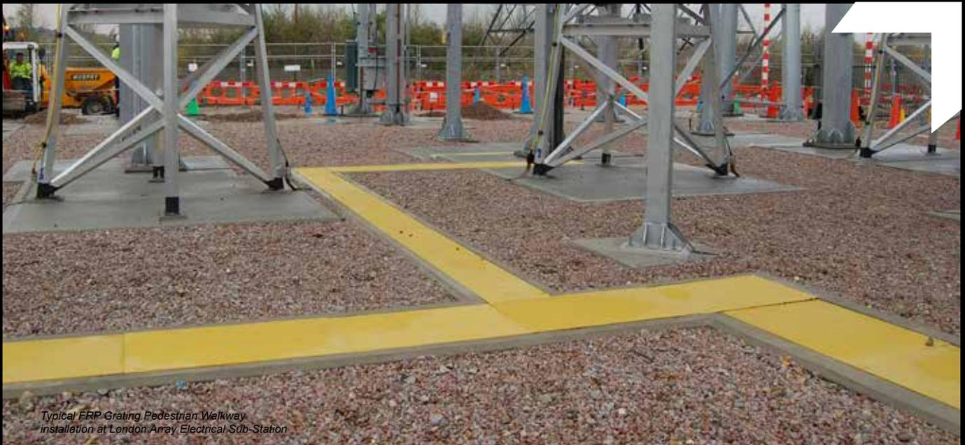
Typical FRP Grating Pedestrian Walkway installation at London Array Electrical Sub-Station
