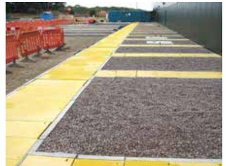
Pultruded through a die, Kite Slab exhibits an incredible strength to weight ratio producing a composite flooring structure that is rigid, strong, lightweight, non-corrosive, durable and maintenance free with an anti-slip surface.
