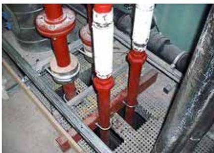
FRP Grating Lift Risers can be installed on each floor during the build to provide worker safety on-site; they can then be cut to suit permanent riser shaft equipment or services
