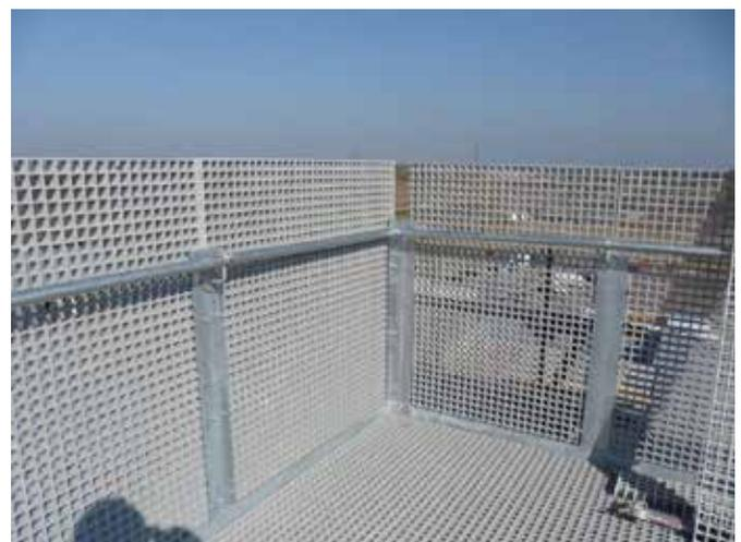
Open grid system ideal to screen items at height and to blend with walkway floor grating
