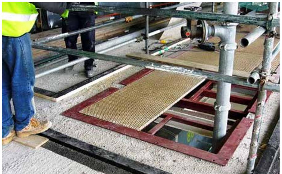
Top of lift shaft fitted with steel frames and fixed within a concrete slab and then decked with Mini Mesh FRP Grating Type 38 Lift Risers to prevent falls and loss of equipment tools during the build process and/or during routine maintenance
