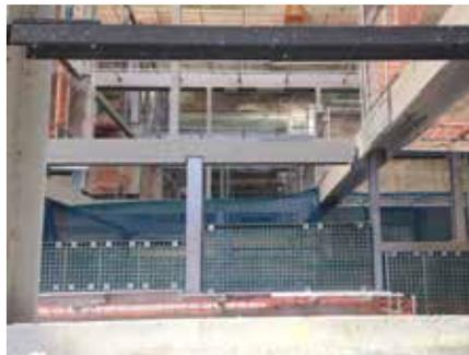
Image showing Mini Mesh FRP Grating Type 38 in place prior to fitment of vertical services which would be cut and reinforced to suit
